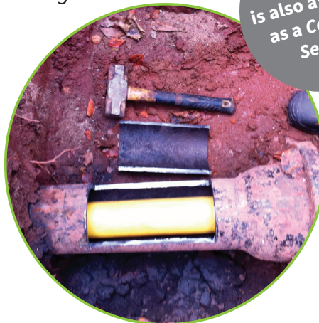
2. Window removed to reveal inserted PE
