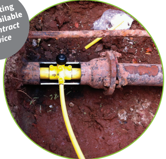
3. Service connections made to the new main
