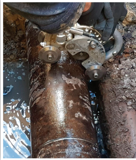
The steel cutter is designed to cut out windows on steel mains to allow the installation of a service top tee where the host main is already inserted with PE. The window is cut out with two semi-circumferential cuts at either end and two longitudinal cuts using a guide frame.
