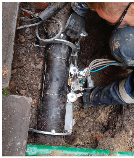
The steel cutter is designed to cut out windows on steel mains to allow the installation of a service top tee where the host main is already inserted with PE. The window is cut out with two semi-circumferential cuts at either end and two longitudinal cuts using a guide frame.
