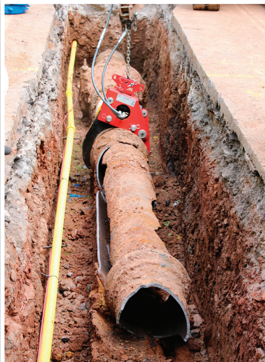
The MACAW cracking a 12" cast iron main
