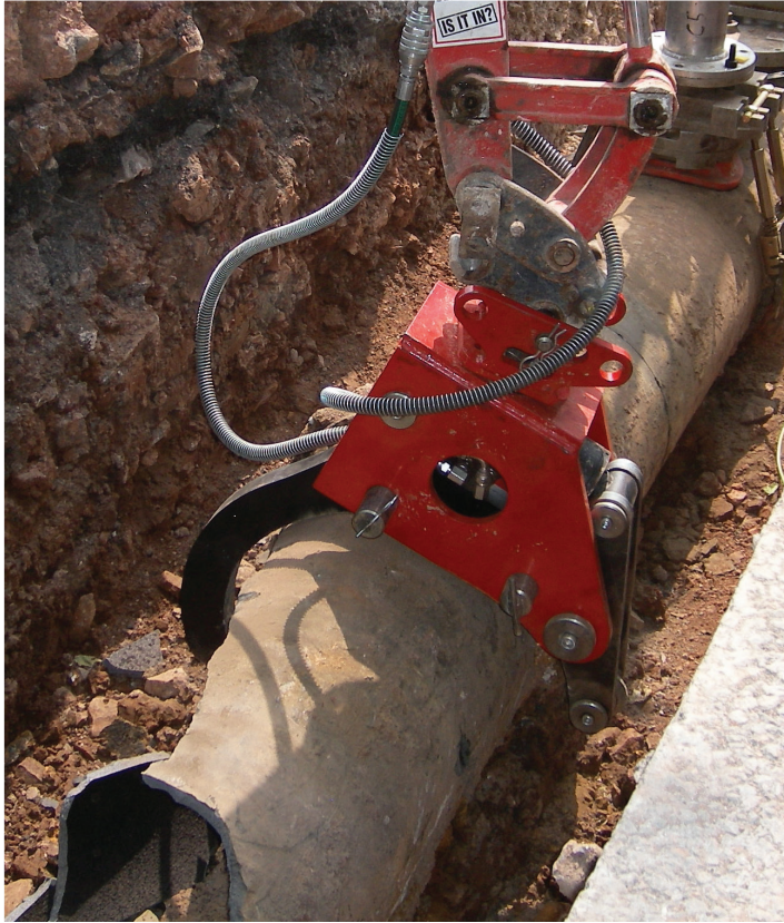
The MACAW cracking a 12" cast iron main
