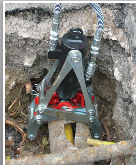
Mini MACAW breaking into a 6" main inserted with 75mm PE
