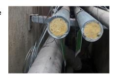
The team leading the project to remove pipework from within an Active Drains Trench was challenged to engineer a solution ensuring C2 conditions were not exceeded. The baseline strategy was to drill holes and inject shaving foam at cut locations along the length of the pipework, enabling the pipework to be safely removed without the danger of creating airborne contamination.
