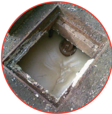
*One of 43 redundant chambers which were filled remotely using expanding polyurethane foam.
