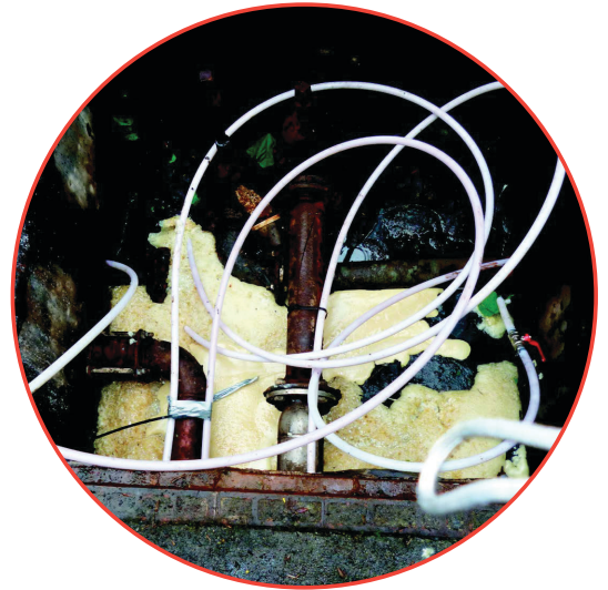
** Access chamber showing where the FOAMBAG's™ were installed in the active drain system, using umbilical line to remotely foam fill entire section.
