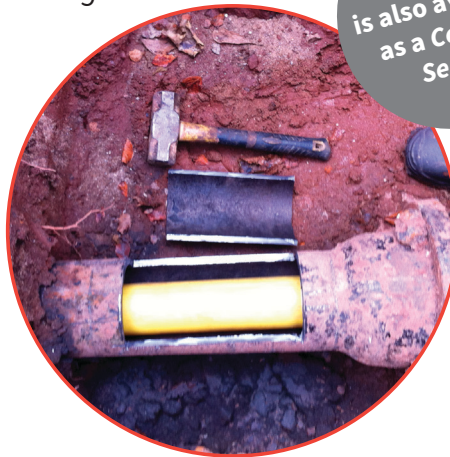
2. Window removed to reveal inserted PE
