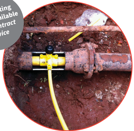
3. Service connections made to the new main
