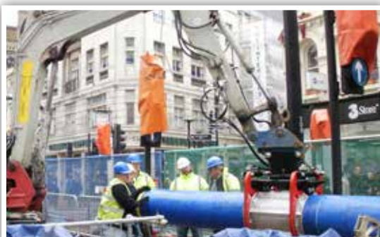
630 Pipe Handler manoeuvring 500mm PE prior to sliplining
