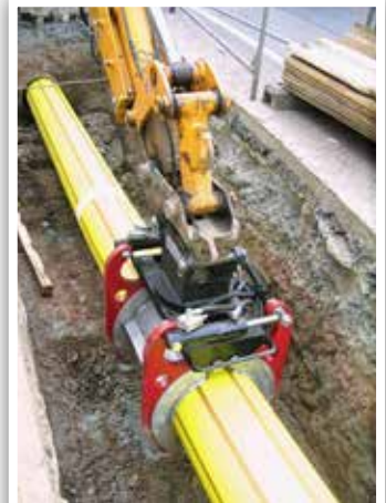
Pipe Handler sliplining 315mm PE into 12" host main
