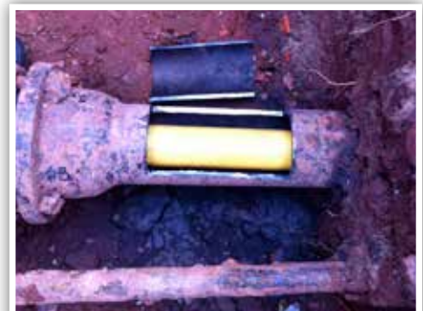
Windows can be cut in a matter of minutes, even on inserted mains
