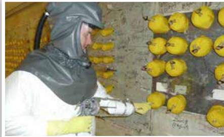
35mm bespoke FOAMBAGs™ installed at the BEPO storage block, Harwell
