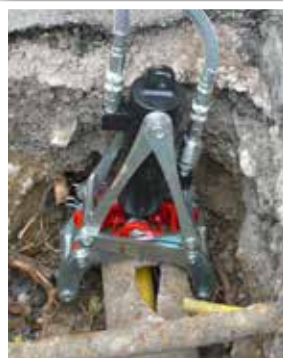
The Mini MACAW breaking a 6" cast iron main inserted with 75mm PE
