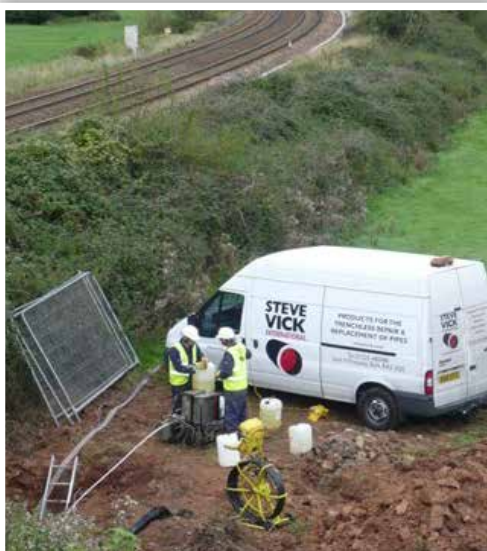
Duct sealing operation carried out on a 10" steel main, under a railway track
