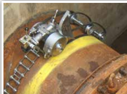
Cutting a 48" cast iron pipe at a water treatment plant
