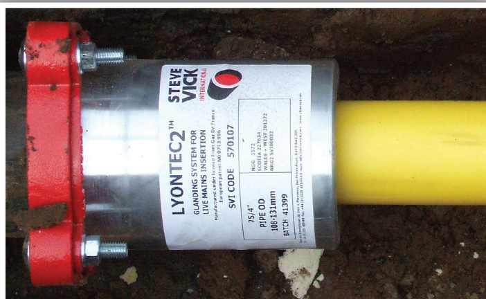
The SVI LYONTEC™ gland box allows insertion of the new PE pipe into the live main in gas controlled conditions
