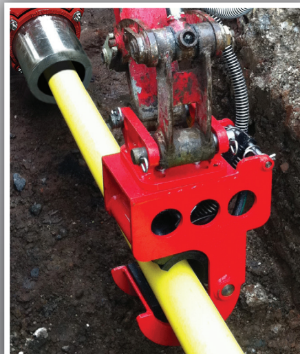
SVI'S range of pipe handling equipment makes pipe insertion safer, faster and more efficient
