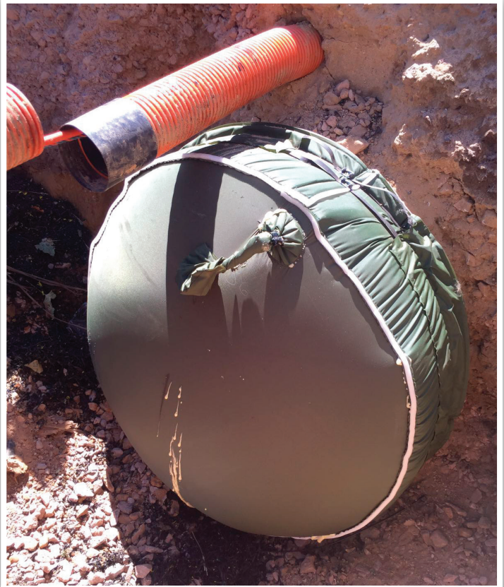
FOAMCAP™ installed on a 24" diameter abandoned cast iron main
