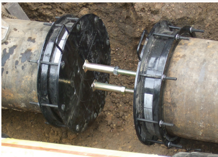
Support Props being used between two end caps
