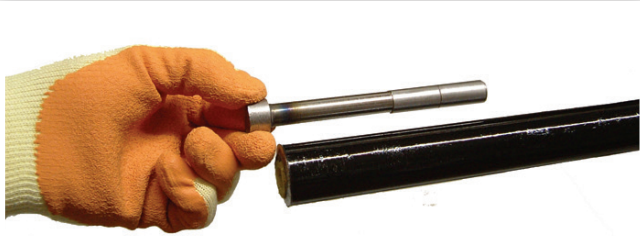
Diagram 1: Using the groove on the Gauging Bar as a guide, the service pipe is scored at the cutting point
