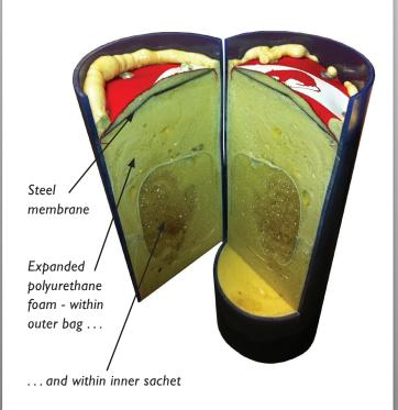
The same pipe, cut in half to show the steel membranes which provide a vermin-proof barrier.
