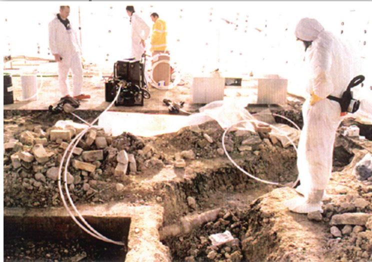
Mass filling redundant fuel lines at Harwell Power Station
