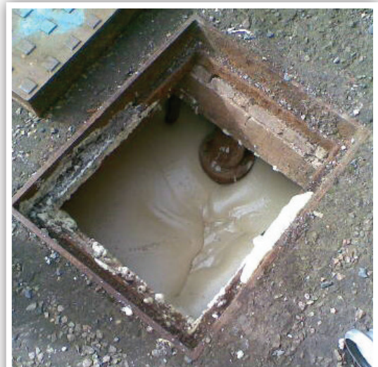
A mass filled chemical drain manhole chamber at Chapelcross Power Station
