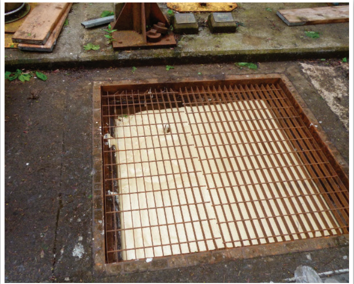
Foam filled manhole chamber with cured foam encapsulating loose debris and sludge
