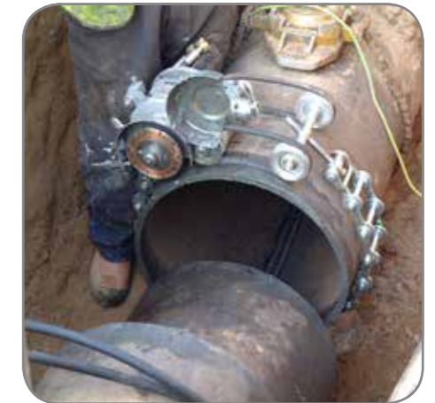
Keel Cutter—Automatic circumferential pipe cutting machine for pipe abandonment and/or diversion
