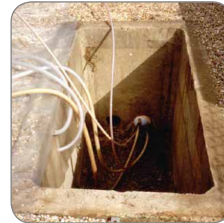
Access chamber showing the cured FOAMBAG™ with umbilical tube in place to foam fill entire length of 180mm pipe
