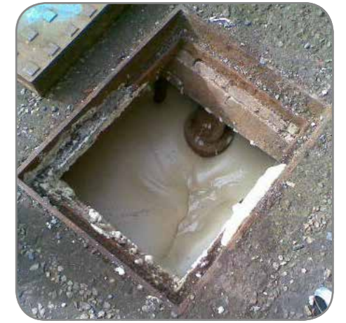
A redundant manhole chamber filled with expanding resin foam. Chapelcross Power Station
