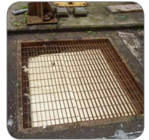
Foam filled manhole chamber with cured foam encapsulating loose debris and sludge
