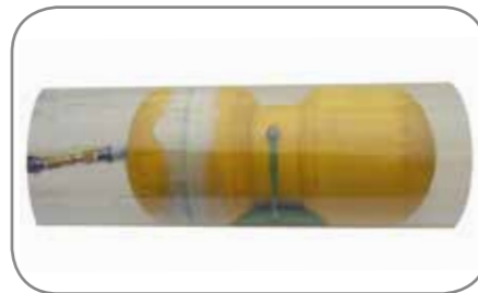
Central void filling with high performance resin via internal injection nozzle
