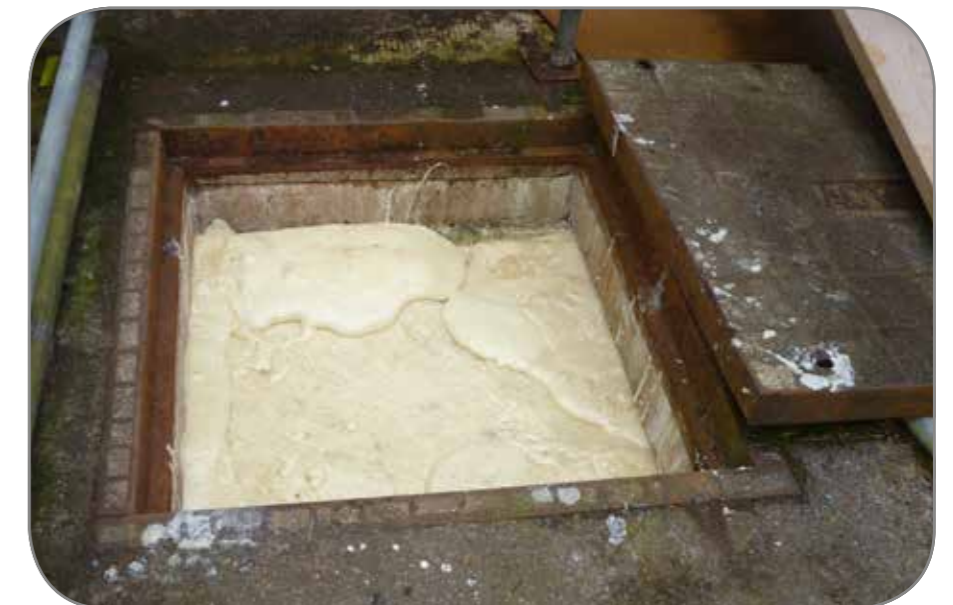
Manhole chamber filled with expanding PU resin foam with bespoke FOAMBAG's™ remotely installed into active drain system below ground.
