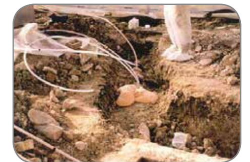
Access chamber showing the cured FOAMBAG™ with umbilical tube in place to foam fill entire length of 180mm pipe
