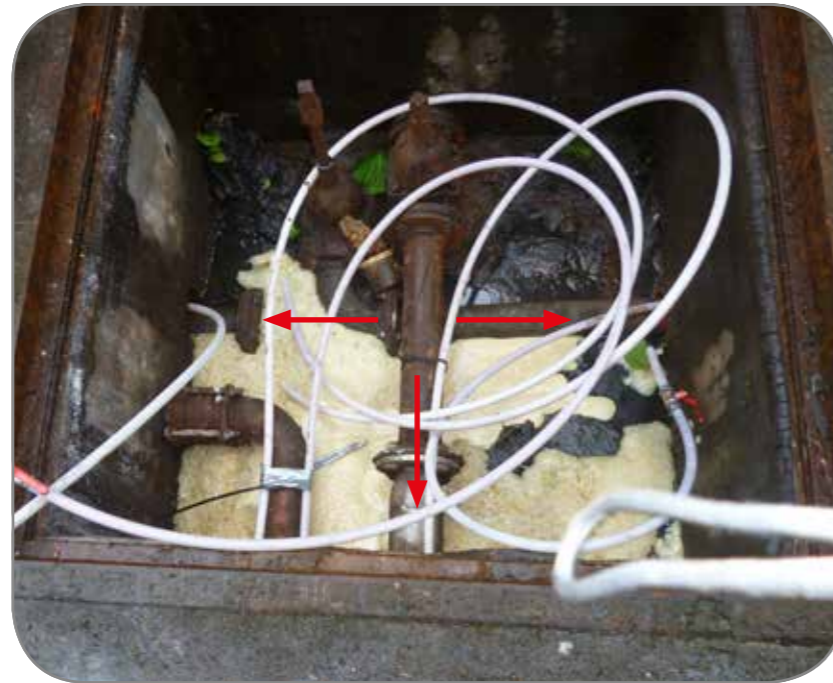
Access chamber showing where the FOAMBAG's™ were installed in the active drain system, using umbilical line to remotely foam fill entire section
