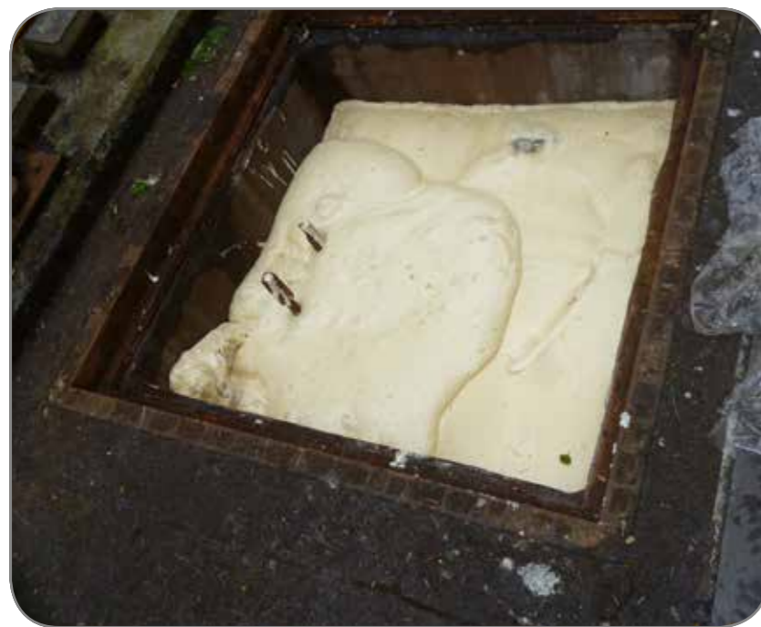
Foam filled manhole chamber
