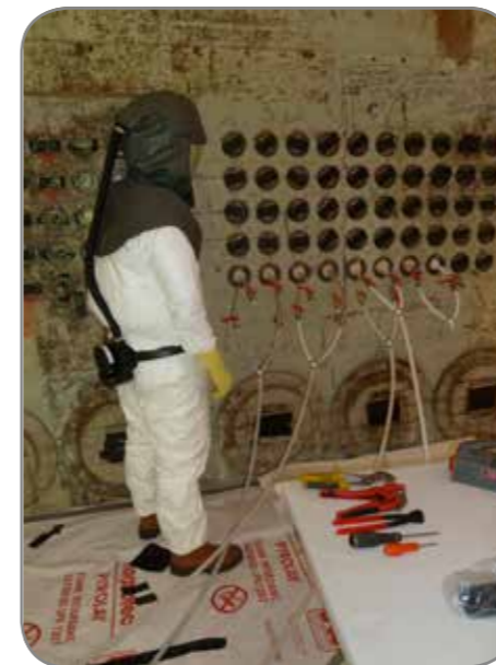
Technicians injecting FOAMSTOP™ bags at the BEPO Storage Block—Harwell
