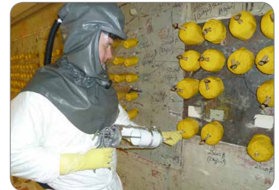
Technicians injecting FOAMSTOP™ bags at the BEPO Storage Block—Harwell
