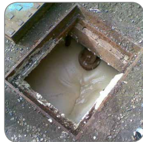
One of the 43 redundant chambers which were filled, remotely, using expanding polyurethane foam
