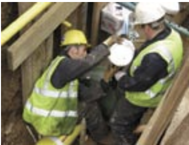
Left: The pre-measured, two-part resin foam is mixed on site and poured into the ENDSEAL™
