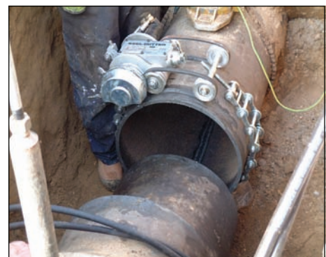
Circumferential pipe cutter
