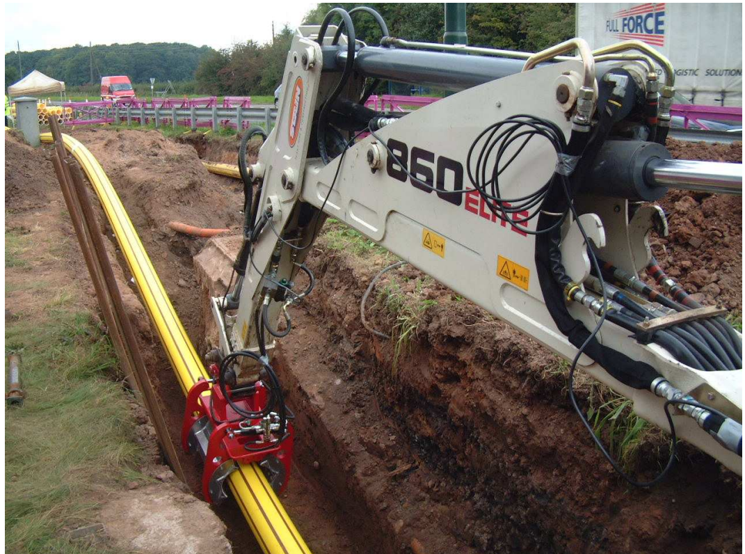
The 355 Pipe Handler fitted with shells inserting 250mm Profuse
