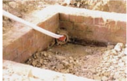
Sealing off underground pipes at a power station
