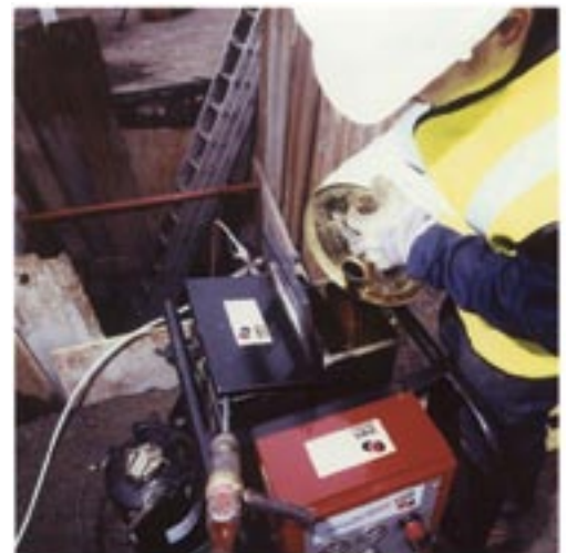
For large diameter 'foam offs', the resin and hardener are mixed and injected using a pneumatically operated machine
