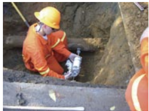
The foam expands to seal the space between the PE and the old main allowing the cast iron to be cut out for service transfer
