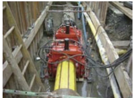
The 630 hydraulic pipe pushing machine
