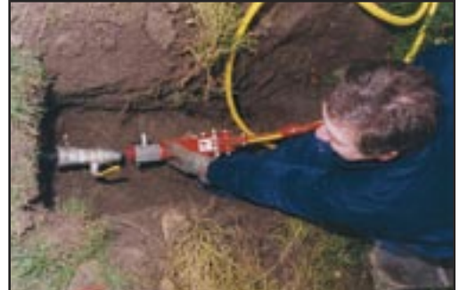
Live gas service insertion allows services to be renewed without excavating in the roadway
