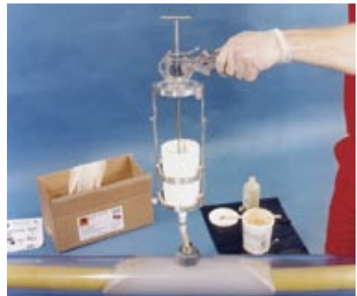
Resin foam is injected into the old main to seal the annular space
