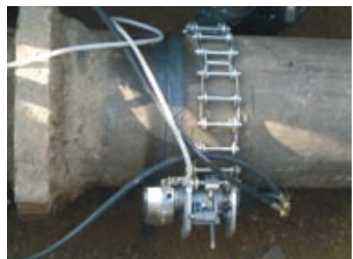
Cutting a 24" cast iron main
