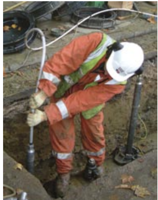
A member of Steve Vick International's Special Contract Services team carrying out a low stopping operation on a large diameter live gas main in 'no gas' conditions
