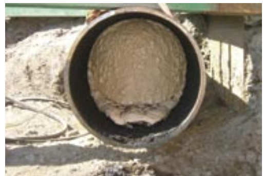
At full expansion, some of the foam seeps through the semi-porous fabric of the FOAMBAG™ to adhere to the wall of the pipe
