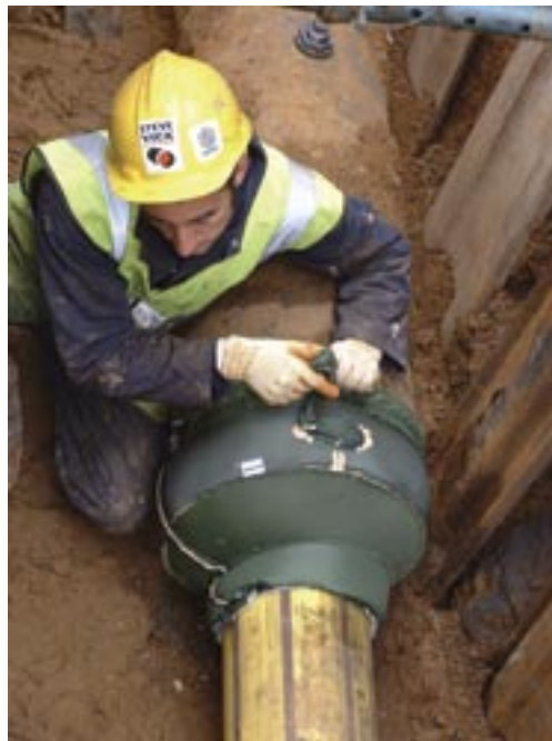
Fitting an ENDSEAL™ on a Live Inserted Main
