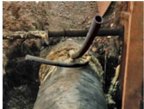
Sealing underground sleeves and ducts prevents the ingress of water or gas
