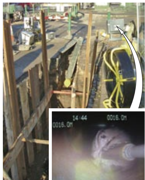
CCTV imaging during a stub end abandonment project
