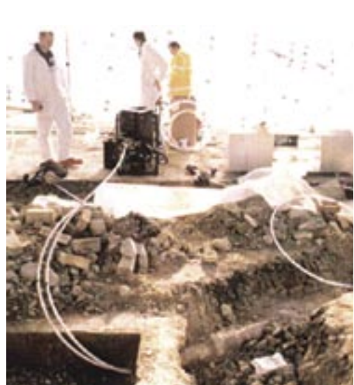
Sealing off redundant underground pipes at a power station
