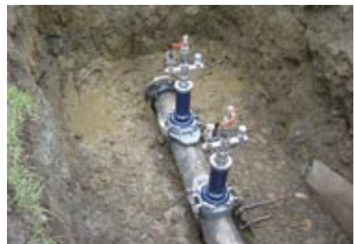
A FOAMBAG™ operation on a medium pressure 6" gas main, Isle of Man.
