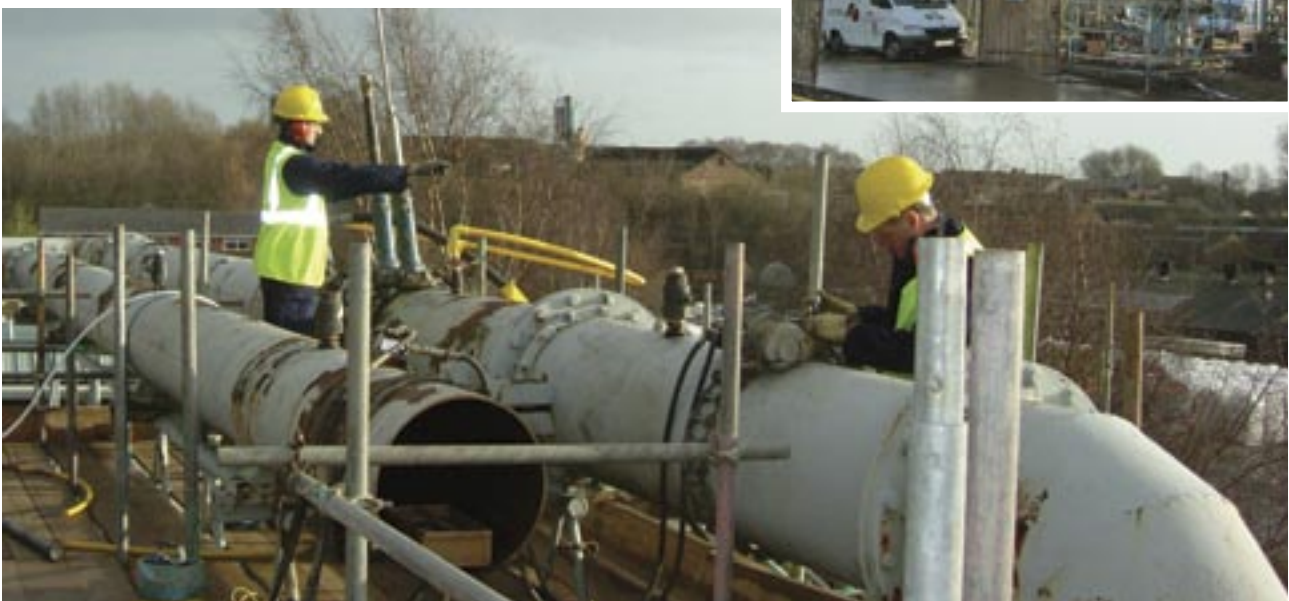
Below and right: Flow stopping 20" and 24" diameter overhead gas mains using expanding polyurethane resin foam and our patented FOAMBAG™ technique, prior to abandonment.
