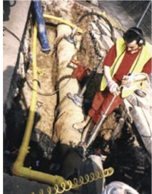
Foaming off a 16" diameter low pressure gas main prior to insertion
