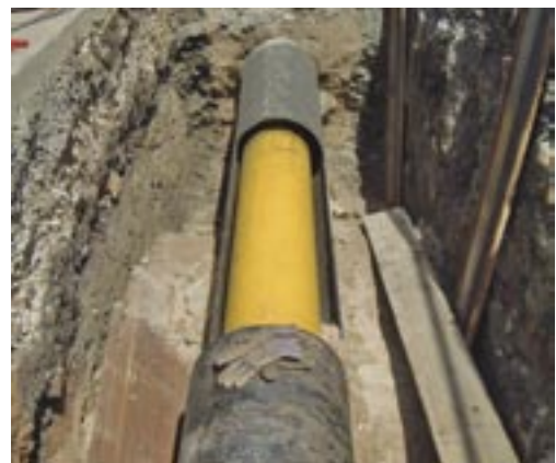
Circumferential and window cutting of cast iron mains
