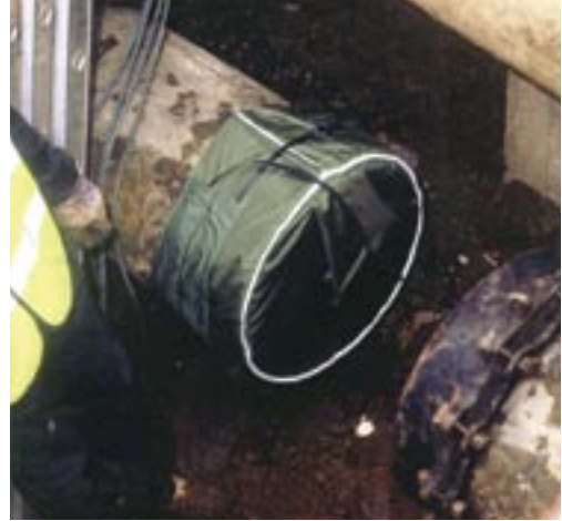
Our FOAMCAP™ system is used to provide a low cost permanent seal on abandoned pipework.
